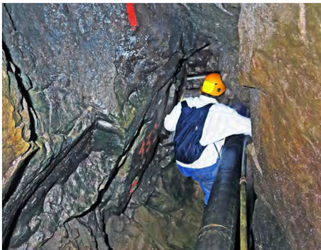
Other sections were rocky, wet and very difficult. Sharing the space with a modern pipeline proved awkward
